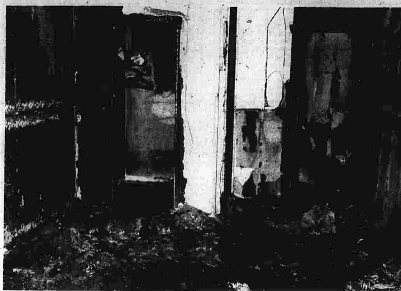
This is the bedroom of an apartment at Falconridge Apartments on New State Rd., gutted by fire this morning.
